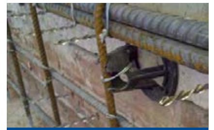
Concrete Shear Wall, Christchurch, NZ DryFix wall tie retrofit
