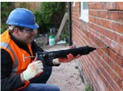
STEP 5 Insert a further bead of HeliBond over the exposed HeliBar, finishing 10-15mm from the face, and 'iron' into the slot using a finger trowel.
