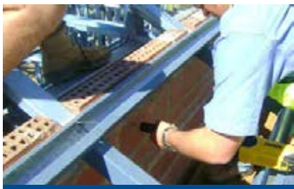
Residential, Western Australia DryFix installation to resist high-wind loading
