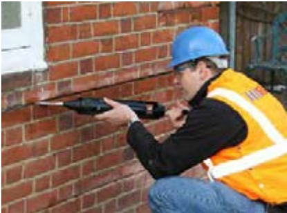
STEP 3 Using a Helifix Pointing Gun, inject a bead of HeliBond to the back of the slot.
