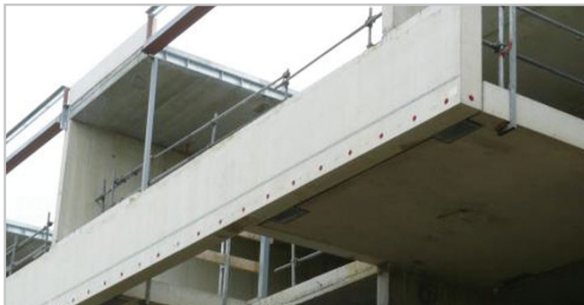
FIXING OF BALCONY RAILINGS
