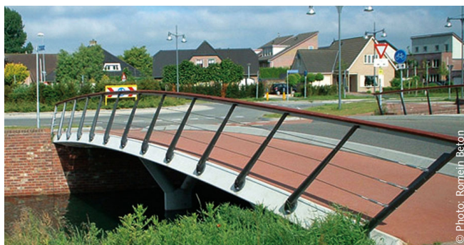
FIXING OF BRIDGE RAILINGS
