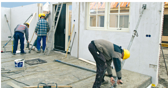
FIXING OF PROPS ON PRECAST ELEMENTS
