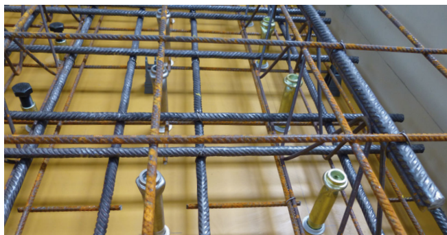
INSTALLATION OF FIXING ANCHORS
