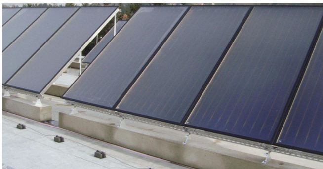
FIXING OF SOLAR PANELS
