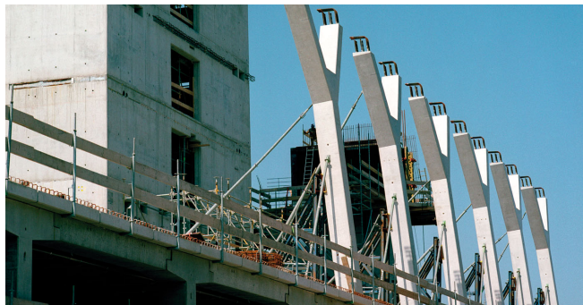
FIXING AND ADJUSTING PRECAST ELEMENTS
