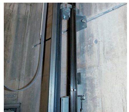
Elevator Guide Rail Connected By Anchor Channel
